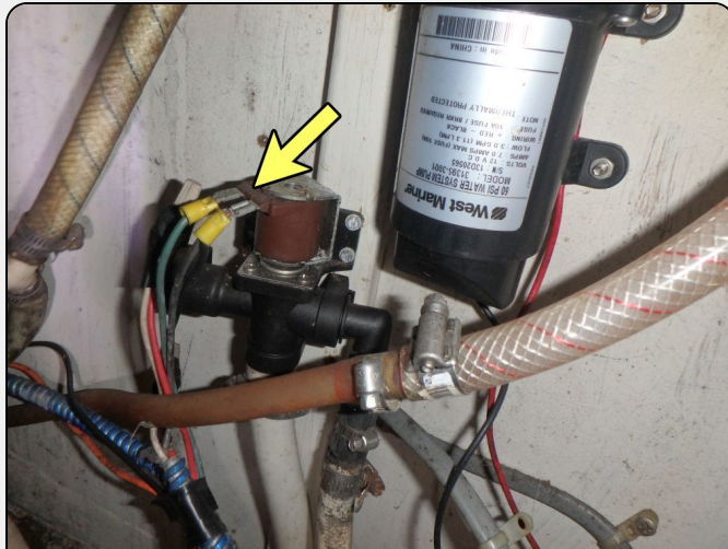
Photo 24: These exposed connectors need to be covered.
