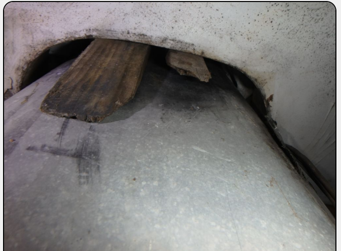
Photo 17: Closer view of the wood shims.
