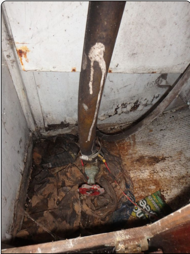
Photo 6 Gate valve in the galley for the sink drain
