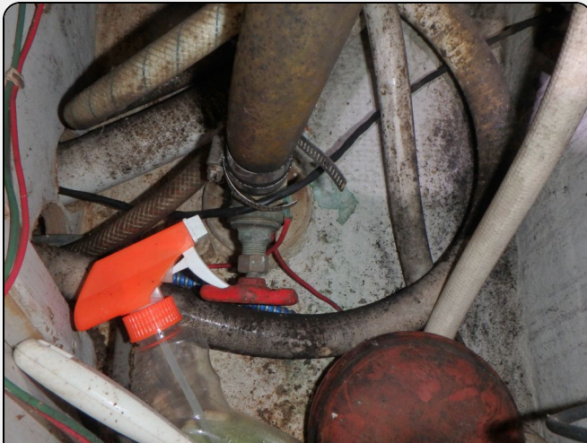
Photo 4: Gate valve in the head - used for the sink drain.
