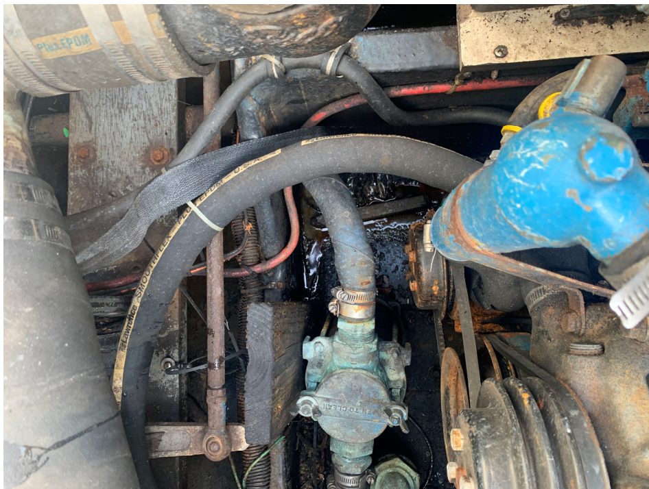
Downward facing view of plumbing and bilge in engine compartment
