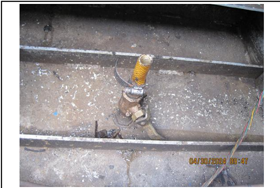
Abandoned raw water intake.
