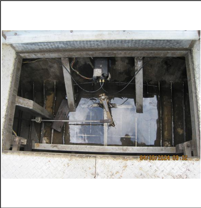
Aft bilge compartment.
